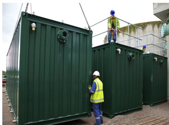
**EP.MBR**.*ffc* Block B plants, can be OPTIONALLY built in Concrete Structure for semi burried or underground installations.
