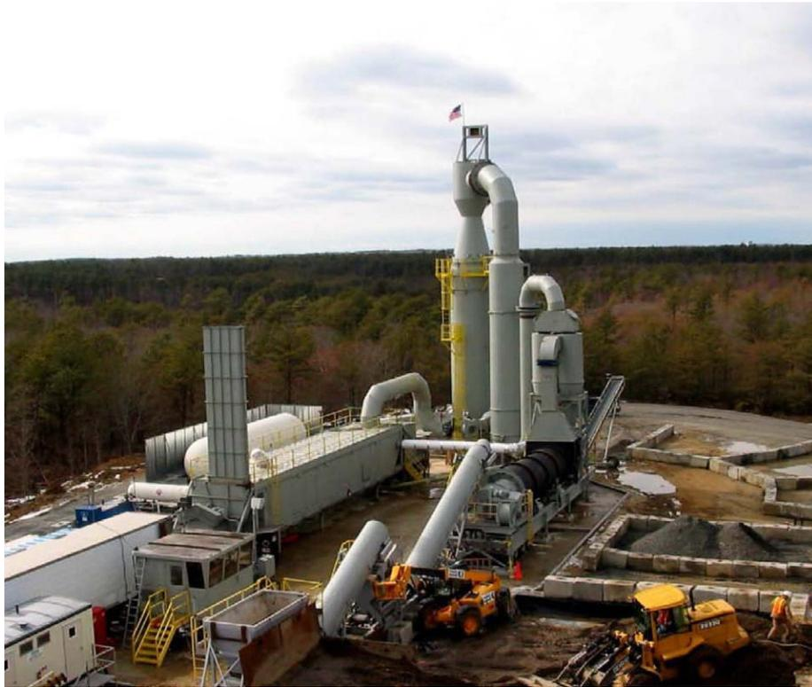
Thermal desorption involves excavating soil or other contaminated material for treatment in a thermal desorber. The desorber may be assembled at the site for onsite treatment, or the material may be transported to an offsite thermal desorption facility. To prepare the soil for treatment, large rocks, debris or metal parts first must be removed or crushed.
