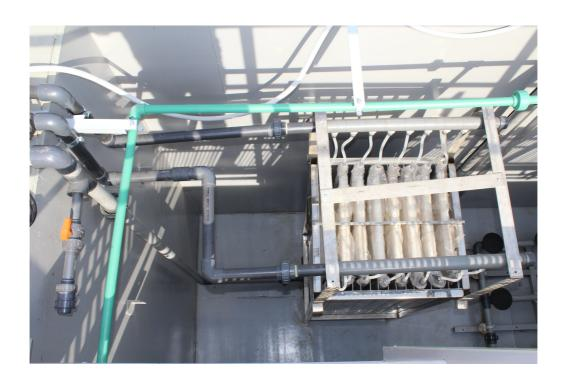
The phase [II] Biological Reactor is working on the Membrane Bioreactors MBR principle which combines the conventional biological activated sludge treatment process with the membrane filtration. Membrane modules are directly immersed in the activated sludge. The activated sludge is separated from membrane modules. Conventional sedimentation processes are not required as the small pores of an ultra filtration membrane separate suspended matter, bacteria, and viruses (pathogens) from the process
